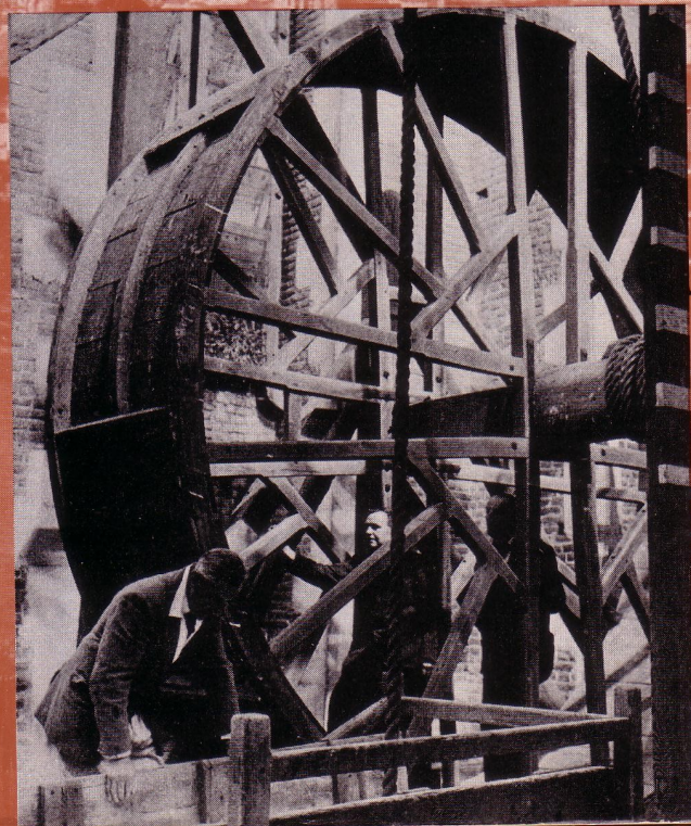
The only way to raise the Hammond Organ to its position over the screen which divides the Nave from the Choir was to use a centuries old treadmill in the Bell Harry Tower.
